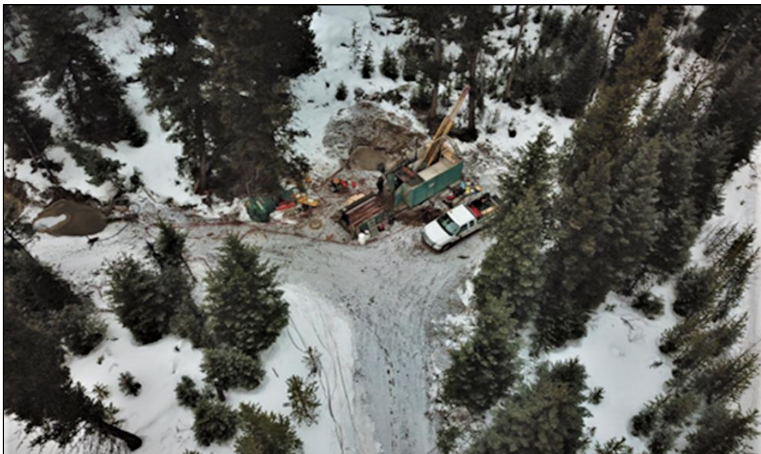
Figure 3: Drone airborne photo of drilling at the Gate/Prime Zone in Fall 2022
